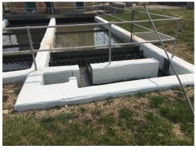
Upon returning the next day, the crew sanded the fiberglass layer to prep the surface for an epoxy topcoat and to remove any fiberglass strands sticking up from the surface. Lastly, a topcoat of Mainstay DS-5 Epoxy was applied to seal the fiberglass system, provide a smooth, continuous surface, and prevent any future concrete deterioration.
