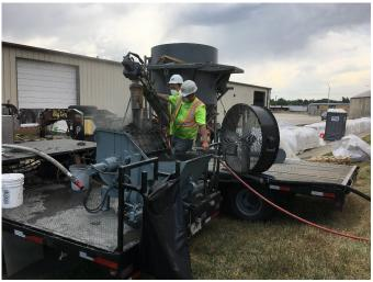
through 1.25" hose for 96 hours nonstop using the robust Madewell Mortar Mixer. The rotor and stator were replaced twice during mortar application due to wear and tear.
