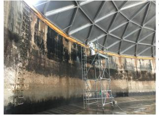
Culy Contracting, Inc. completed a project for the City of Longmont in Colorado that utilized over 2,500 bags of Mainstay ML-72 Sprayable Microsilica Restoration Mortar. A crucial concrete equalization basin at the City's wastewater treatment plant had experienced severe corrosion due to high levels of hydrogen sulfide gases. To repair the structure, Culy was contracted to apply 1.5" of Mainstay ML-72 to approximately 10,000 SF of the basin's concrete walls.
