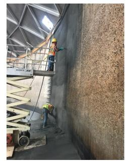
Mainstay ML-72 mortar was applied in 6-foot-wide sections at 1.5" thick using Madewell shotcrete equipment and scissor lifts. Each section was dampened with water prior to mortar application. The mortar was hand troweled smooth and broom finished to achieve a slightly textured surface. After finishing, a water-based concrete sealer was applied to prevent cracking.
