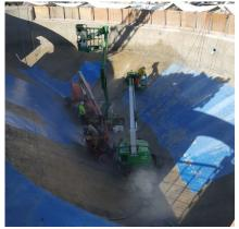
To begin, Thomarios performed high pressure water blasting at 40,000 psi. This surface preparation method was employed to completely remove the old coating and roughen up the underlying concrete to achieve a substrate suitable for mortar application.
